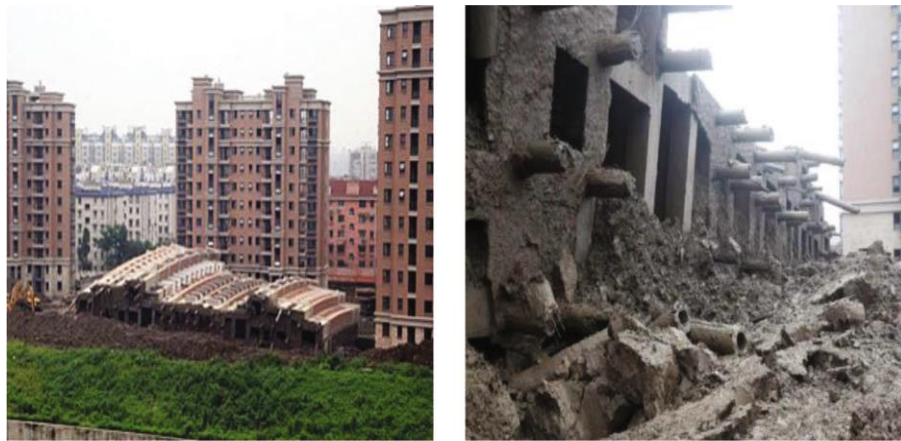
Figure 7: Collapsed high-rise apartment building—result of improper construction
