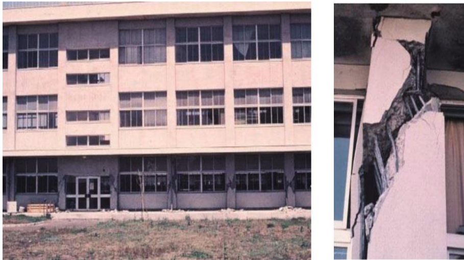
Figure 6: School building in Hachinohe, Japan damaged during 1968 Tokachi-oki earthquake (Aoyama, 2010)
