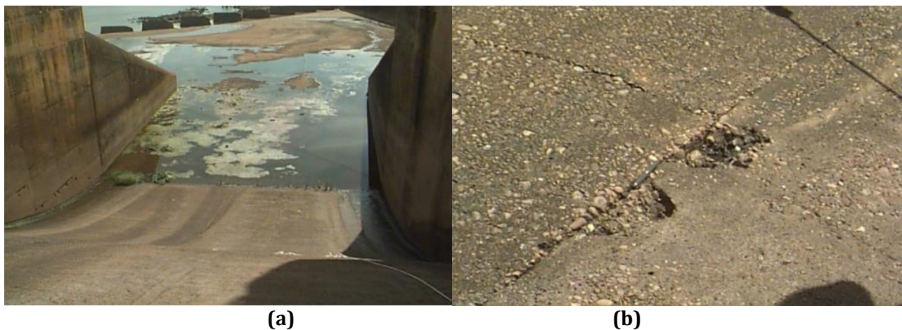
Fig. 2: (a) Spillway dam presented deterioration by abrasion. (b) Defects in the concrete structure caused by abrasive process (Galvão, 2012)
