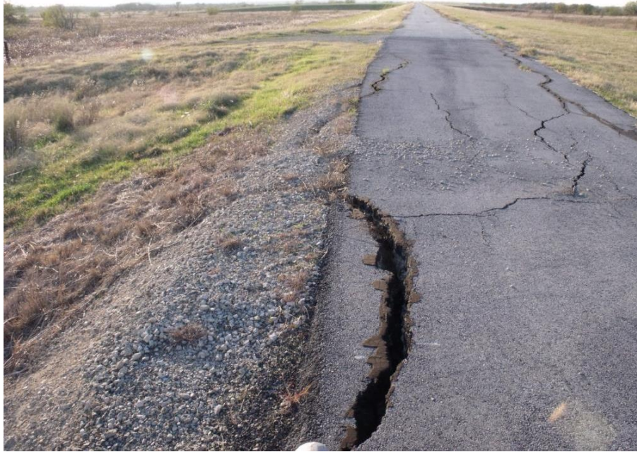
Fig. 3: Typical cracking on Lewisville Lake Dam with clear signs of aging (Adamo, 2020).
